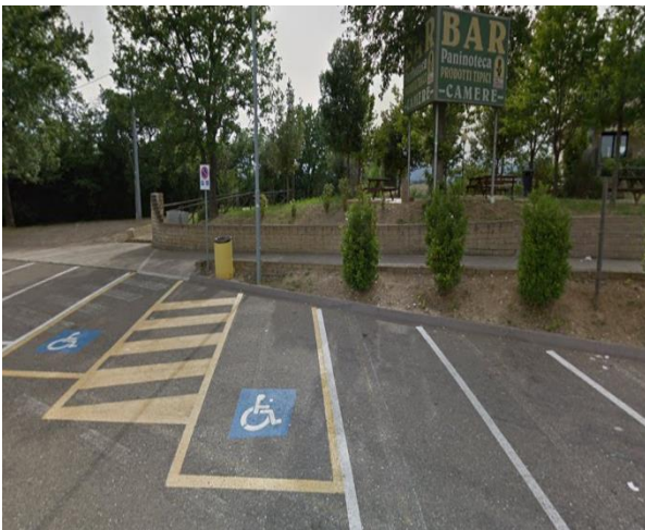
60 parking and ramp for terrace entrance
