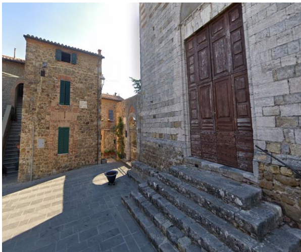
166 Entrance portal with steps
