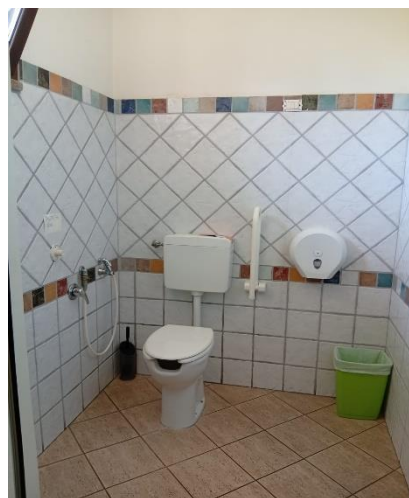
67 Toilet with grab bar
